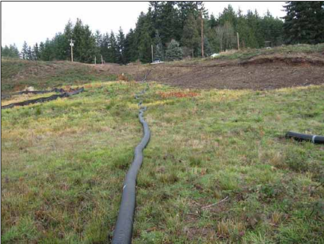
Photo 18. Reach 4. Myricks Fork in 6 inch pipe.
