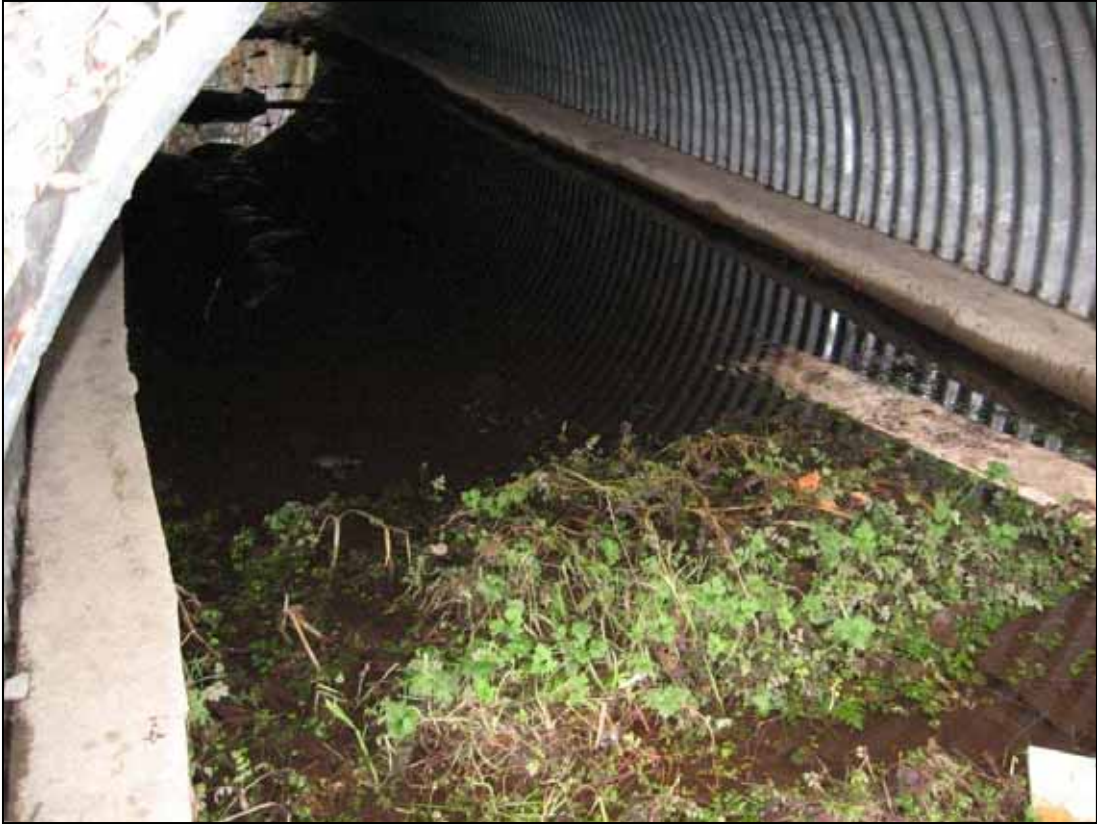
Photo 14. Reach 8. Myricks Fork through 12 ft culvert.
